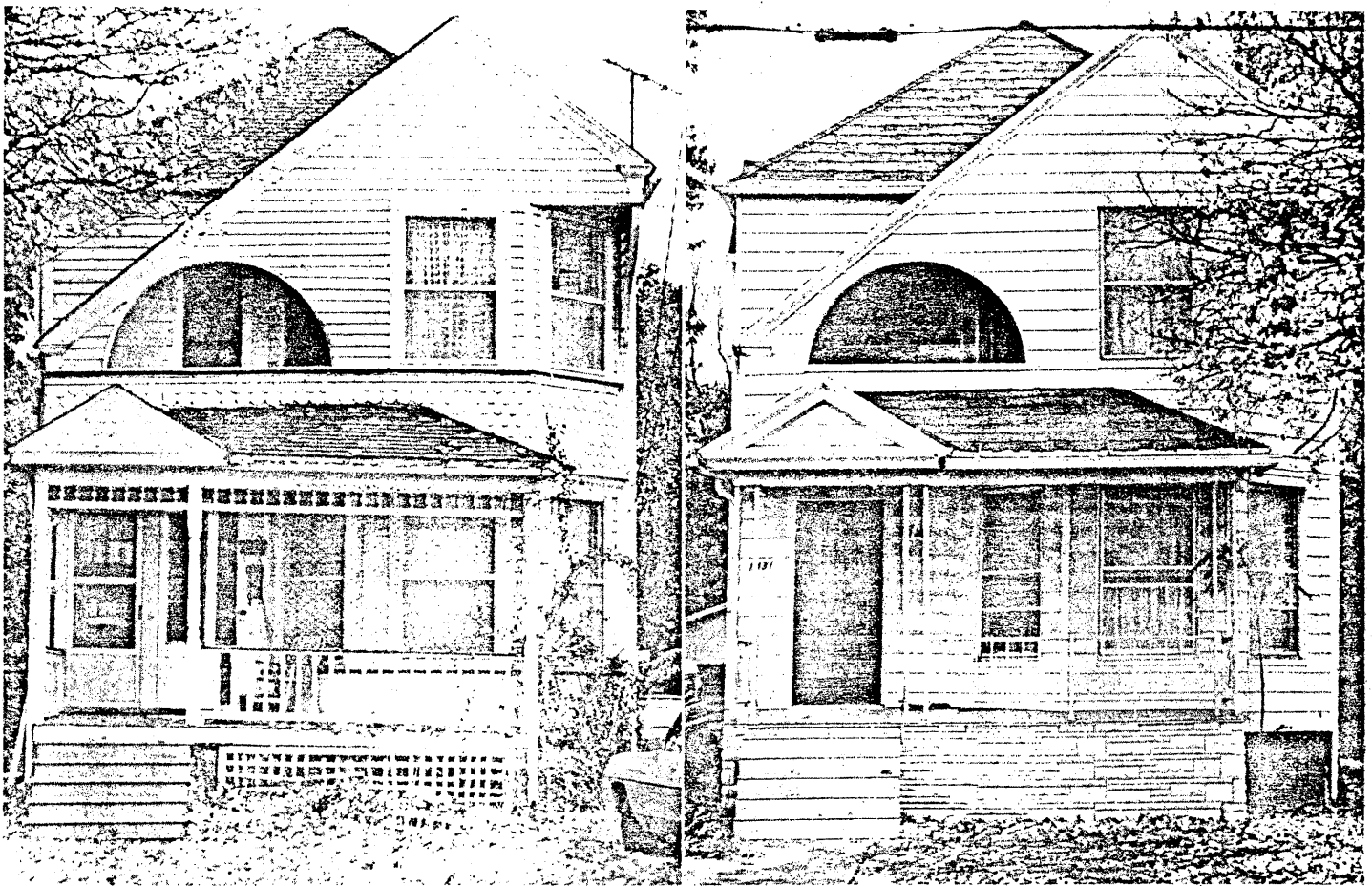
These houses were identical until the one on the right was covered with aluminum siding. Though the houses do not possess high architectural significance, they did have character and visual interest. The house on the right lost its character and visual interest when the variety of textures and details were covered with aluminum siding.
