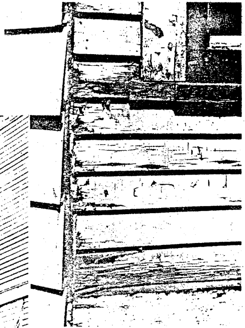
Above: Each strip of aluminum siding covered more than two original clapboards, changing the original character of the house. This photo also shows how the windowsills had been cut away to accommodate the synthetic siding.
