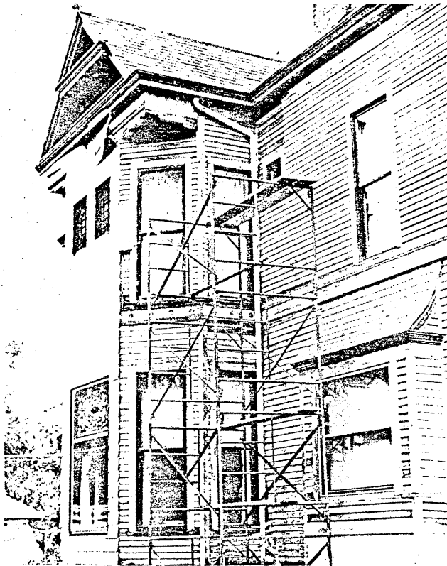
Above: As the aluminum siding was removed, it became evident that water had been seeping behind the siding and that the clapboards beneath had rotted. As a result, all clapboards above the second-floor windows had to be replaced. Water had also collected at the raised banding below the second floor windows, rotting the clapboards there. Note the shadowlines of the bull's-eye details that were removed to accommodate the siding.
