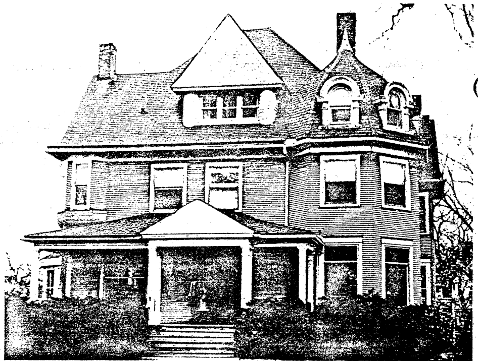
Below: During the restoration project, the aluminum siding was removed, exposing missing or damaged clapboards and trim. Note the delicate bowing of the turret, which was obscured by the aluminum siding. The wood elements will be repaired as necessary, and the house will be painted.
