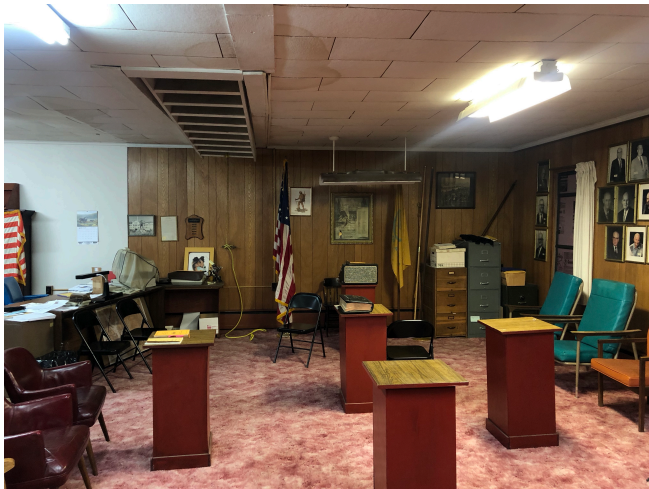
Fluorescent lighting fixtures in the Meeting Room
