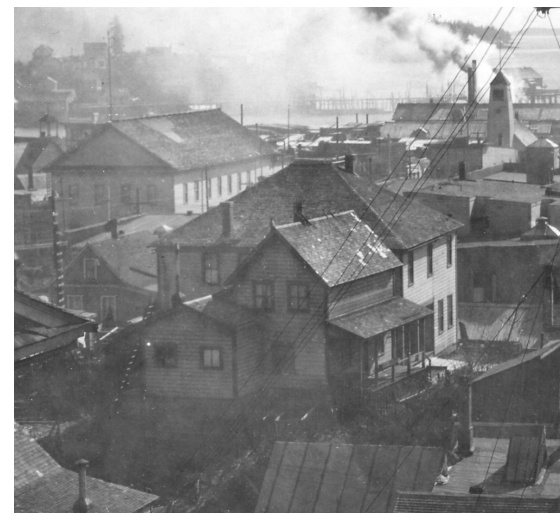
This c. 1913 photo shows the partially-obscured features of the original exterior including the many double-hung windows, hip roof and its then still visually prominent location. In spite of changes over its 121-year history, its basic features and many of its original trim details could be restored.
