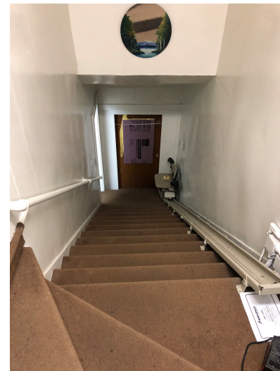
A photo taken by the survey team of the primary access from the main floor to the second floor meeting room and apartment. A stair lift serves as the only means of accessibility for Pioneer members with limited mobility.
