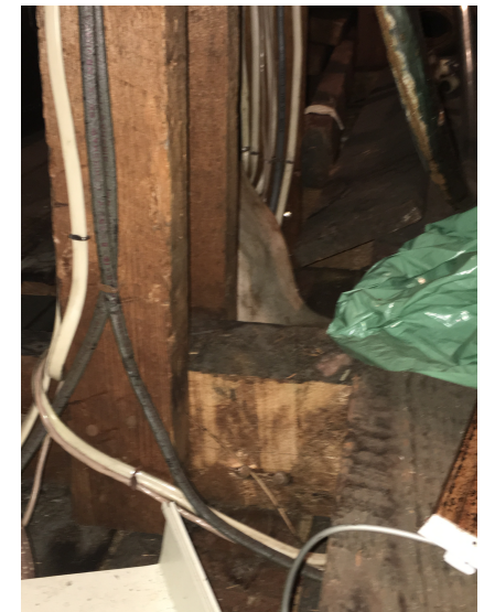
Beam/stud configuration in attic
