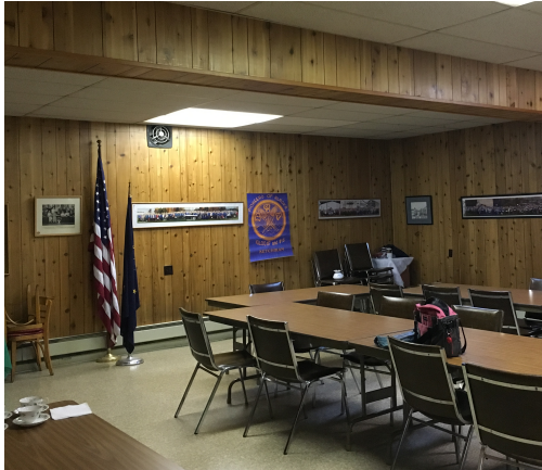
Support beam in Hall for 2nd Floor
