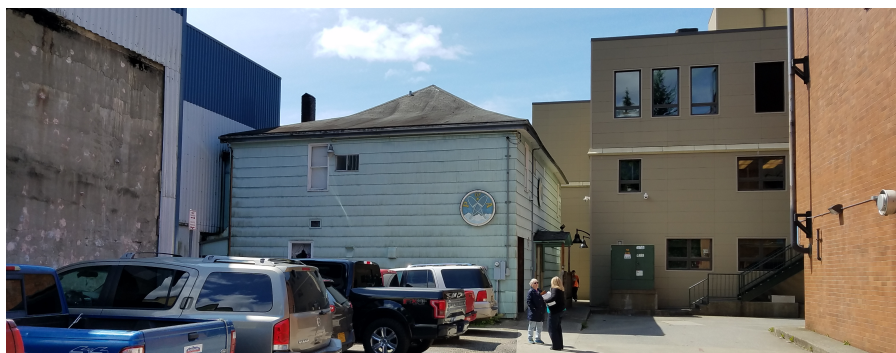
The Pioneer Hall is today surrounded by other buildings and its constrained site creates challenges for occupancies, occupant loads and exits.
