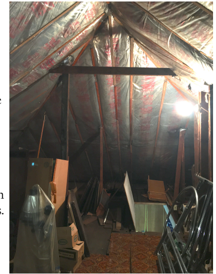
Rafter configuration in attic
