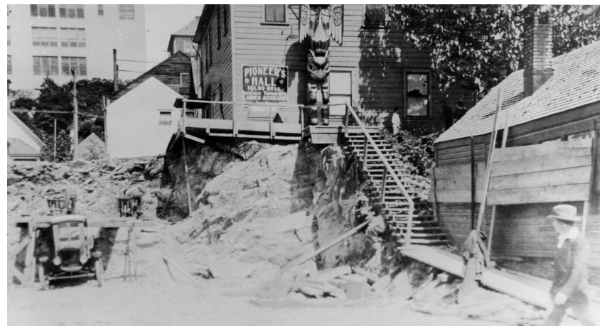
Later in 1925, the "Pioneer's Hall" sign was added as well as a new covered entry on the NW elevation (Pioneer Way). The original double-hung windows and channel siding are evident in both photos.
