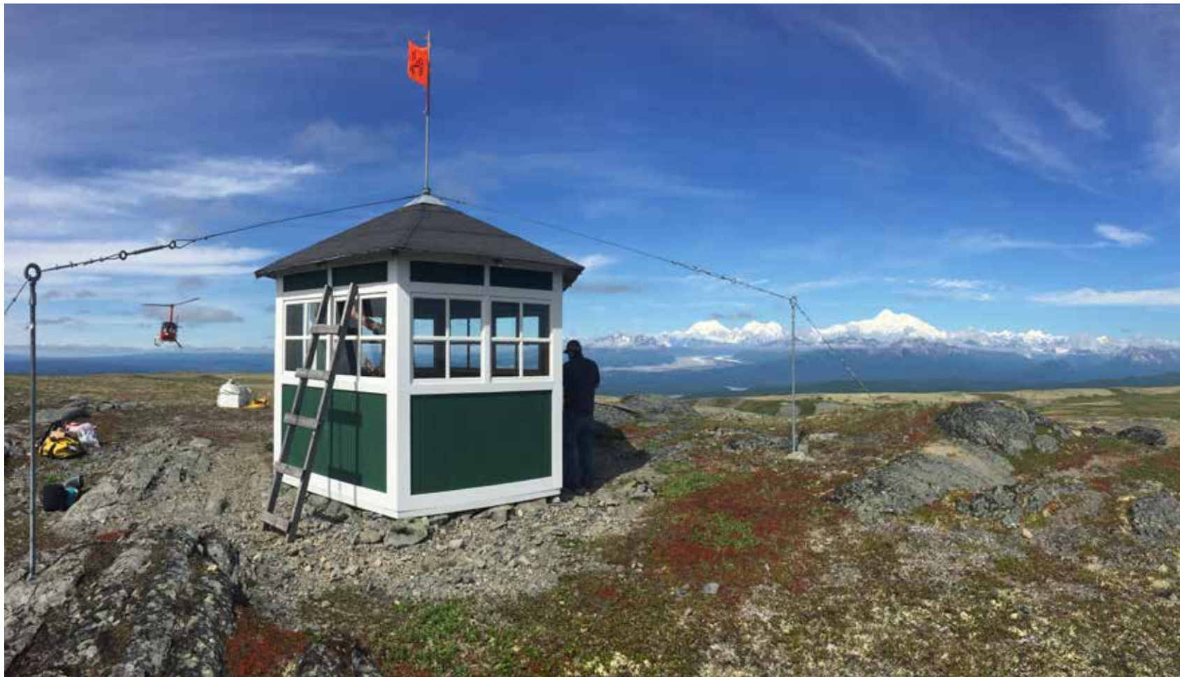
Curry Lookout rehabilitation, Denali State Park. (OHA photo)
