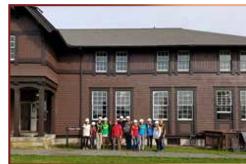
Whitmore Hall facade rehabilitation, Sheldon Jackson School NHL. (Alaska Arts Southeast photo)
