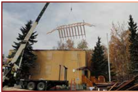
Pioneer Schoolhouse roof replacement (Kristine Bunnell photo)
