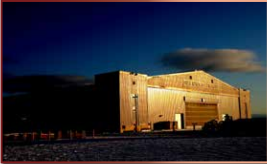
Hanger I, Ladd Field NHL, Fort Wainwright, Fairbanks. (Fort Wainwright Cultural Resource Division photo)
