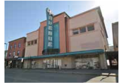
4th Avenue Theater-Anchorage
