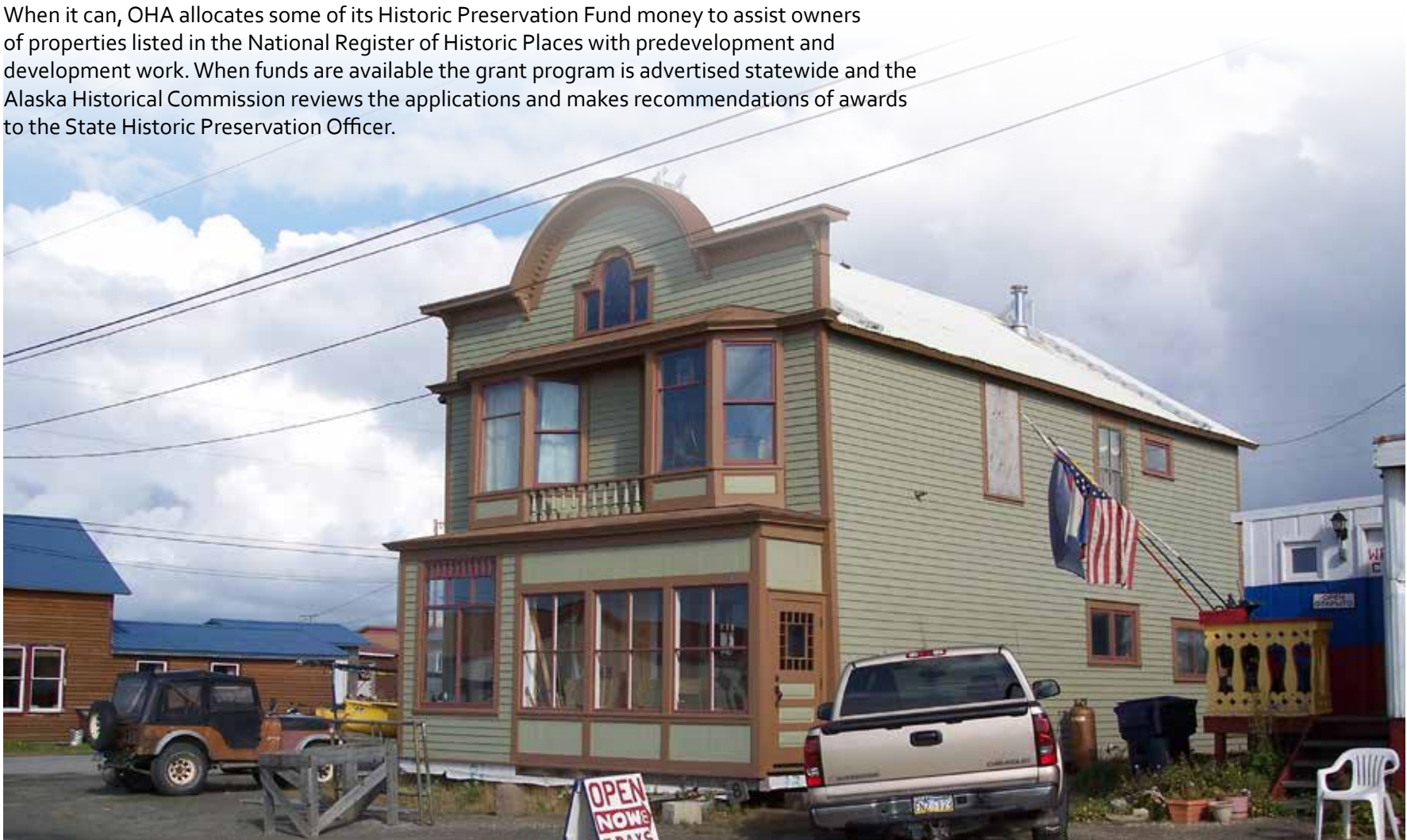
Discovery Saloon, HPF funded exterior rehabilitation project 2012, Nome (OHA photo)
