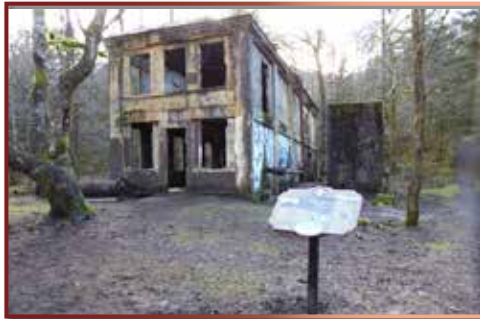
Interpretive sign, office building at Treadwell Mine. (Gary Gillette)
